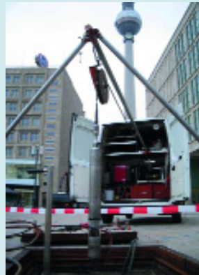
Filter pipe inside a well.
