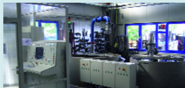
Pump test stand. Reproduced with kind permission of Würdig Pumpentechnik, Berlin
